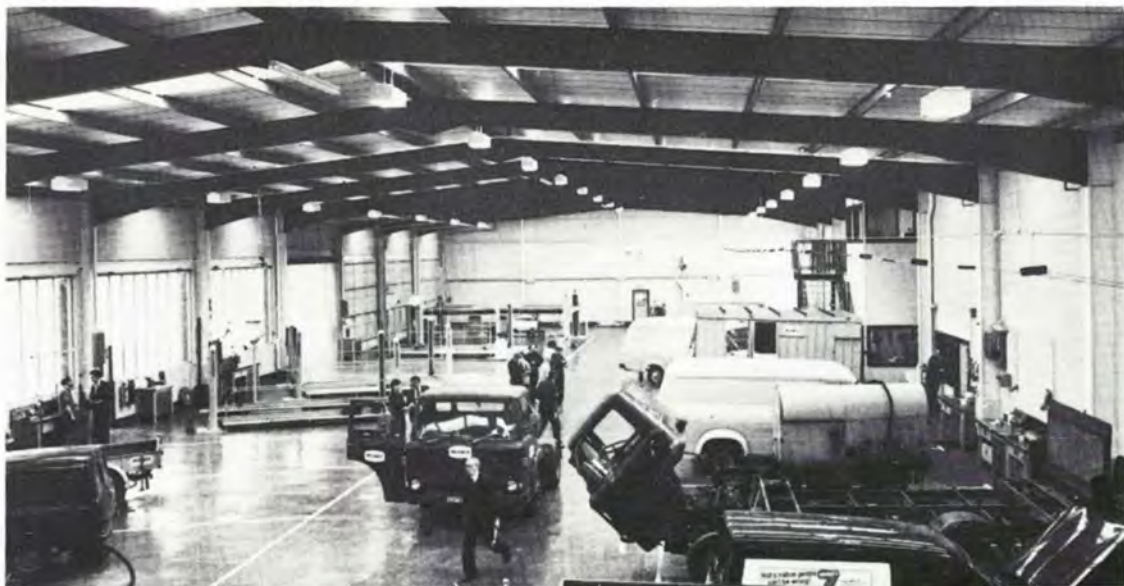
Activity inside the new garage at Lister Drive.
